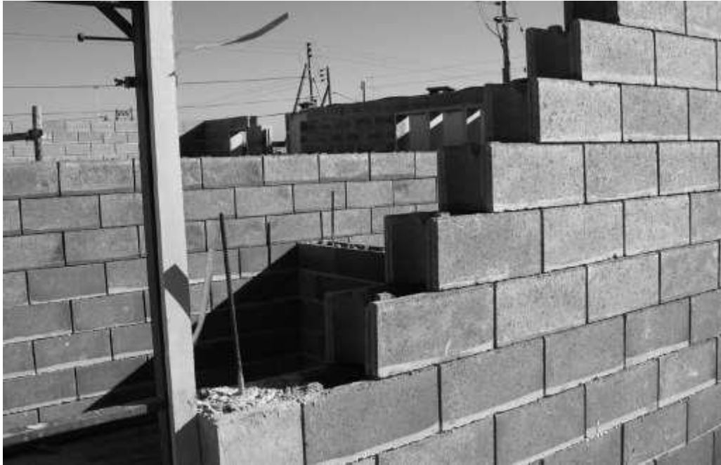
Fig. 6 Hollow Concrete Block Wall
