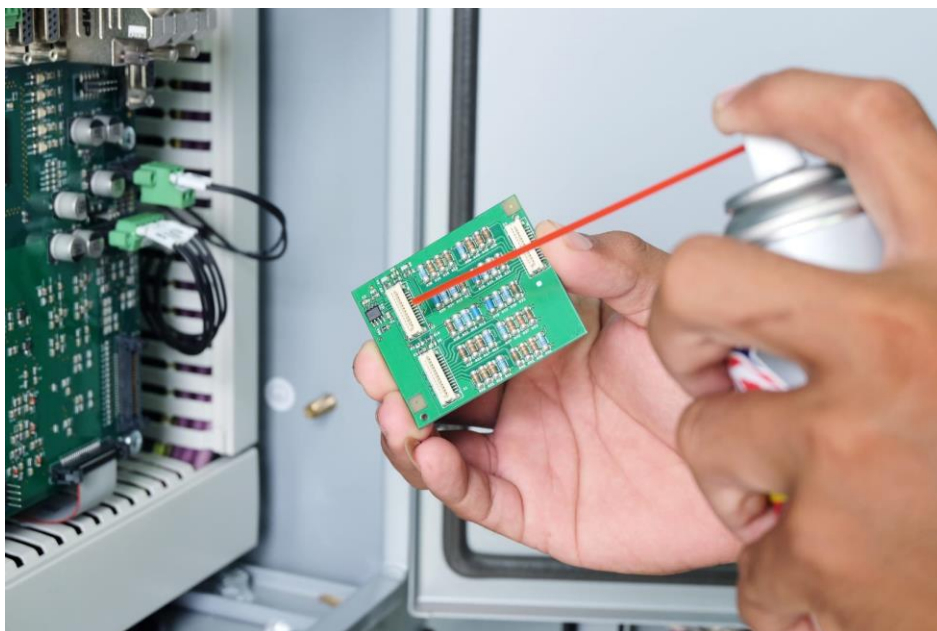
Fig.5:Cleaning the PCB
