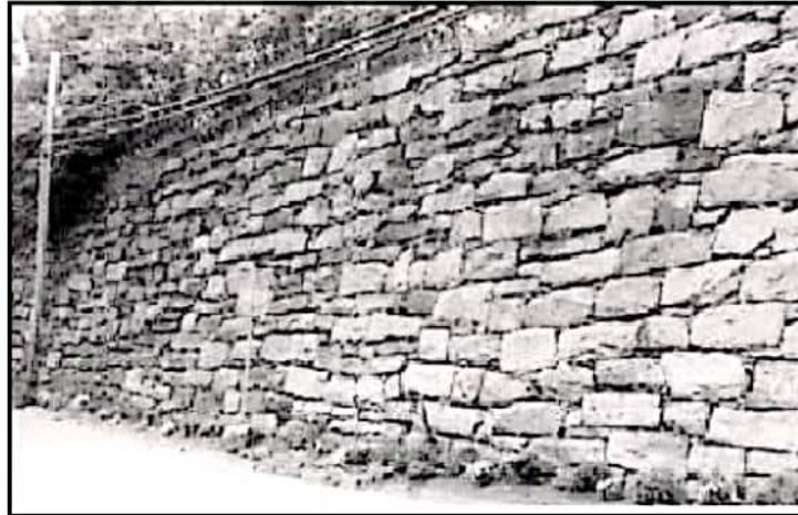
Fig 6.2 Dry Stone Gravity Wall
