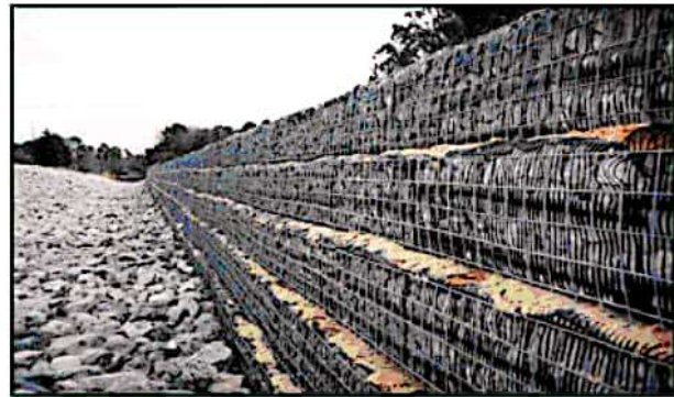
Fig.6.9 (ii) Gabion Wall
