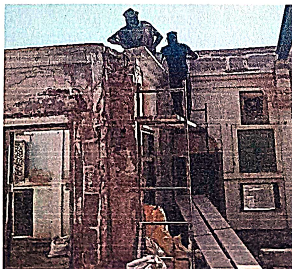
Fig. 4.5 wall of Haveli
